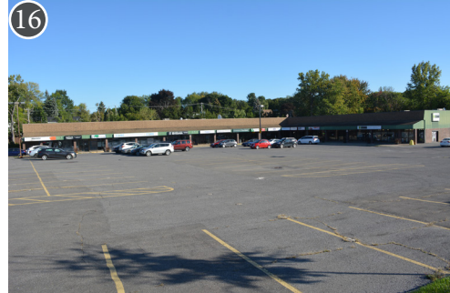
16- Centre commercial de Beaconsfield
